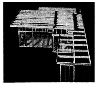
Fig.3. R.M. Schindler, Mrs. George Harris House, Los Angeles 1942-44. Framing model, scale 1'=1'-0", constructed by DalTech students July 1998.
