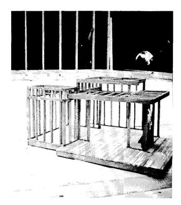
Fig.6. Rudy's Cabana framing model, scale 1"=1'-0", constructed by DalTech students July 1998, on site with cabana framing in progress.
