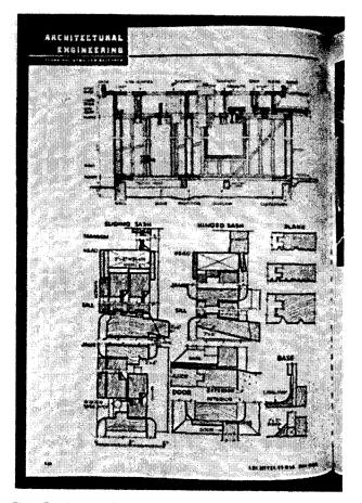
Fig. 1: Framing conditions and typical details as published by Schindler in the "The Schindler Frame," *Architectural Record*, May 1947.
