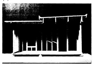
Fig.2. Schindler Frame sampler model, scale 1"=1'-0", constructed by DalTech students July 1998.
