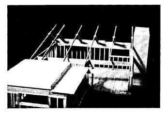
Fig.4. R.M. Schindler, Felix Presburger House, Studio City 1945-47. Framing model, scale 1"=1"-0", constructed by DalTech students July 1998.
